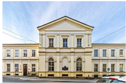
Library and Study Room, U Nemocnice 4, Praha 2
